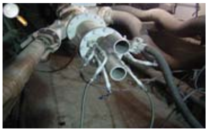
A burner for petcoke, solid wastes (two channels), liquid wastes/heavy fuel oil ( http://www.dynamis-ma.com/ ).
